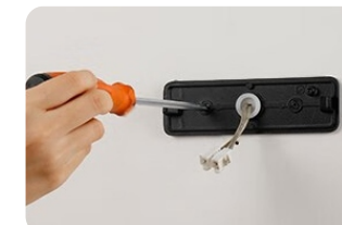
2. Secure the hanging plate in the mounting position
