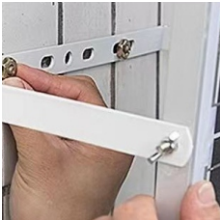
Align the hole in the light holder with the wall nail
