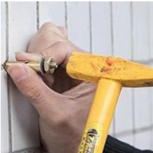
Hammer the wall nails in place
