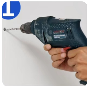
Drill the wall to be placed with a drill
